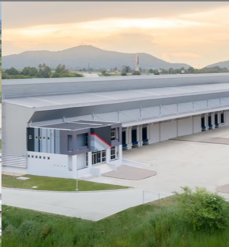
Ready-built Warehouse Logistics Park
