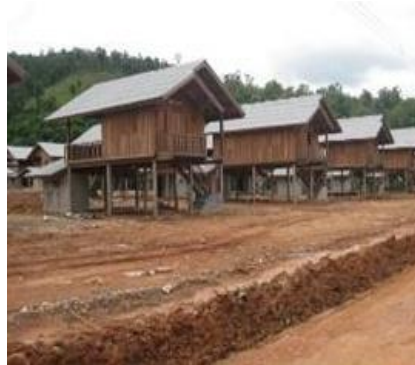
RAP: Complete resettlement house for villagers
