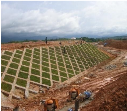
Power plant area: Slope paving (pre-construction work)
