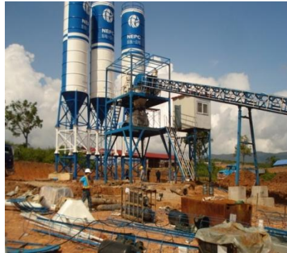
Power plant area: Cement silo for power plant construction
